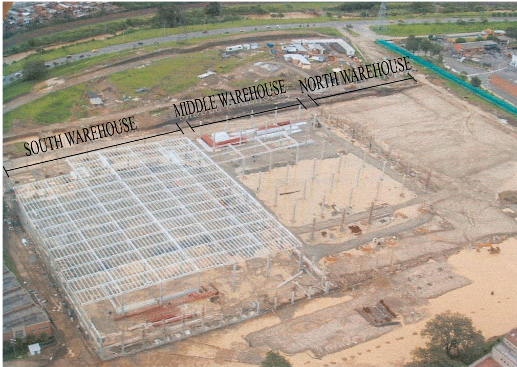
Picture 1 – Distribution Center during the initial construction (Notes: 1. The middle and north warehouses were destroyed by the big fire. 2. For dimensions see figure 1)
