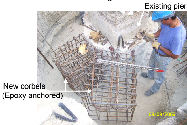
Figure 16. Epoxy anchoring of the reinforcement for the new corbels
