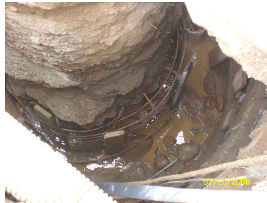
Figure 15. Placing of the new bell reinforcement
