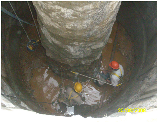
Figure 14. Construction of bell enlargement
