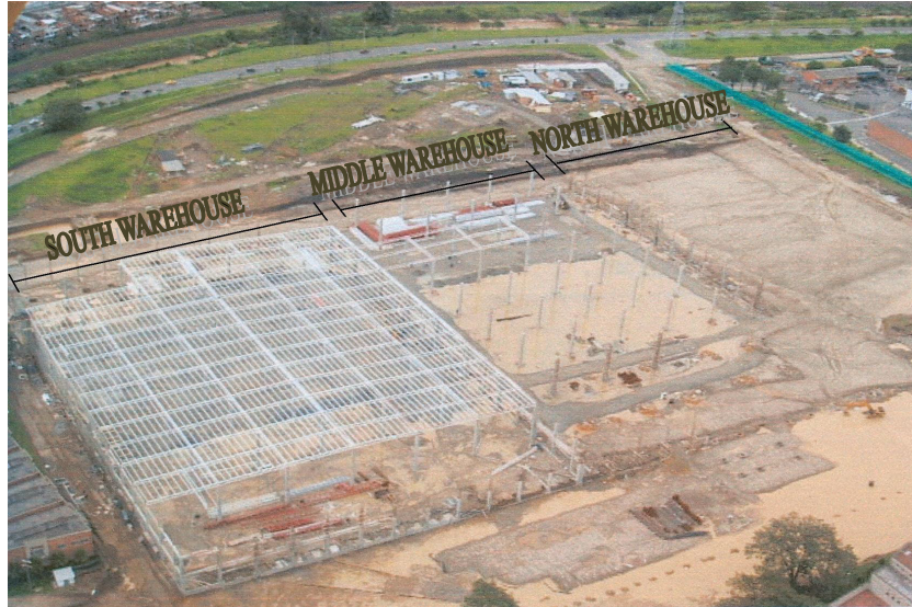
Figure 1. Distribution Center during the initial construction (Notes: 1. the middle and north warehouses were destroyed by the big fire. 2. For dimensions see figures 3, 4)
