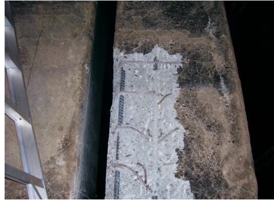
Figure 8. Taken of samples of steel for laboratory testing
