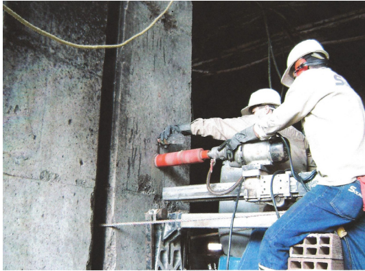
Figure 7. Extracting concrete cores
