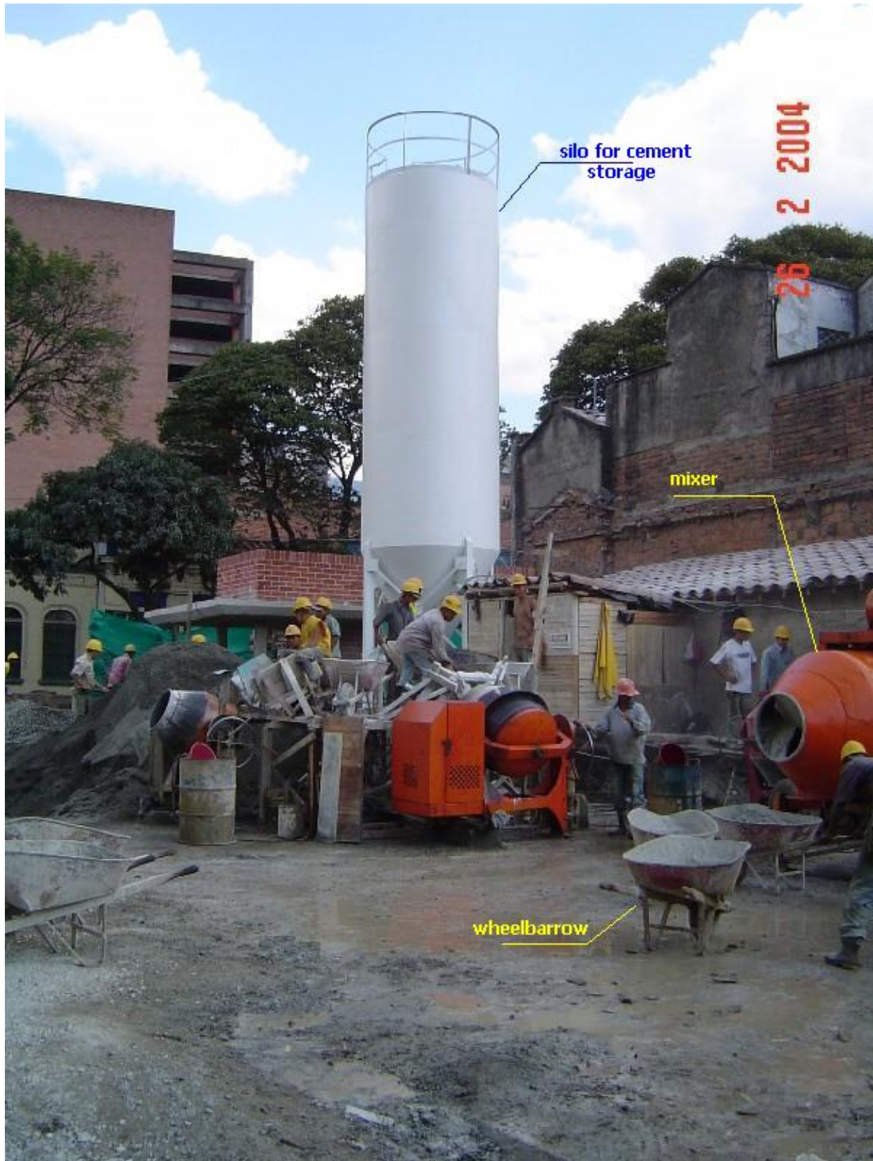
Figure 5a. Concrete producer plant on building site. OPTIMA S.A. construction project.
