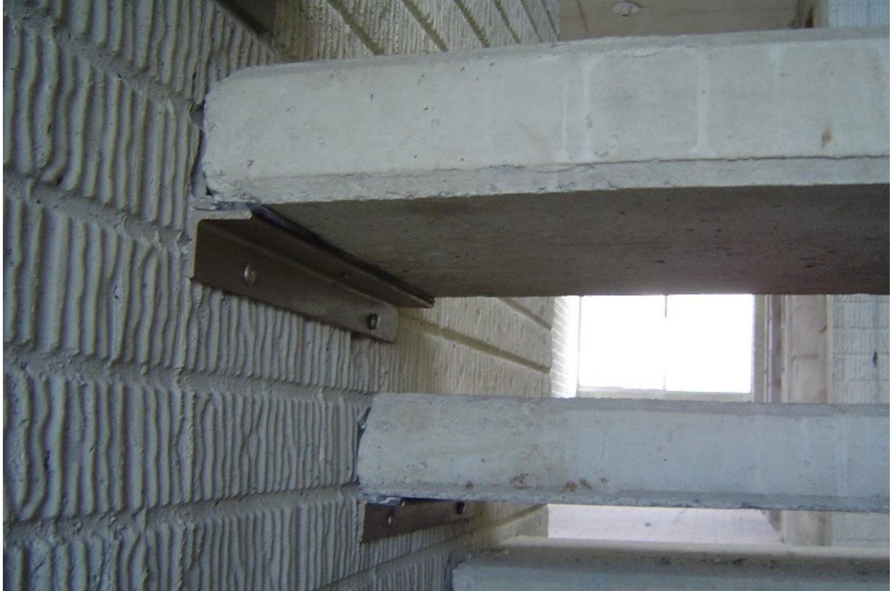
Figure 7. Precast stair supports. OPTIMA S.A. construction project.
