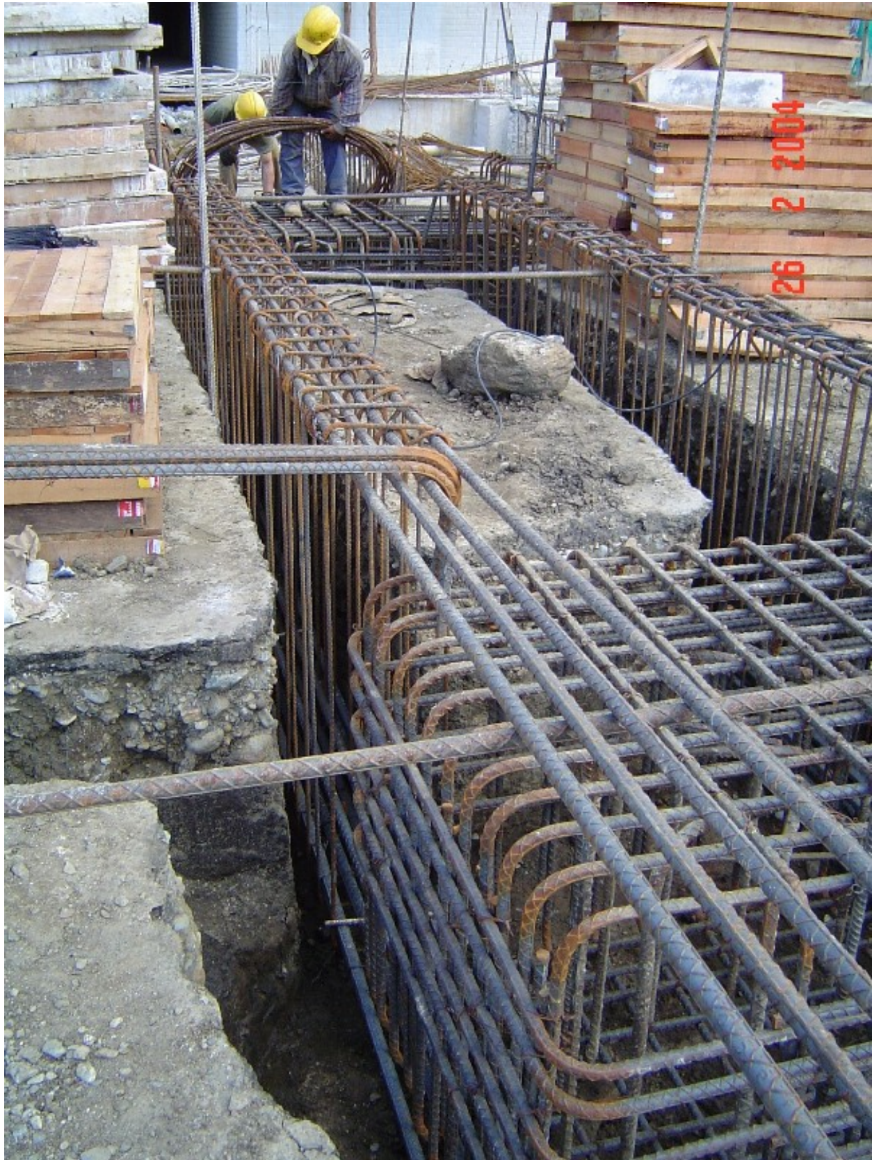
Figure 6b. Perspective view of the reinforcement foundation beams. OPTIMA S.A. construction project.
