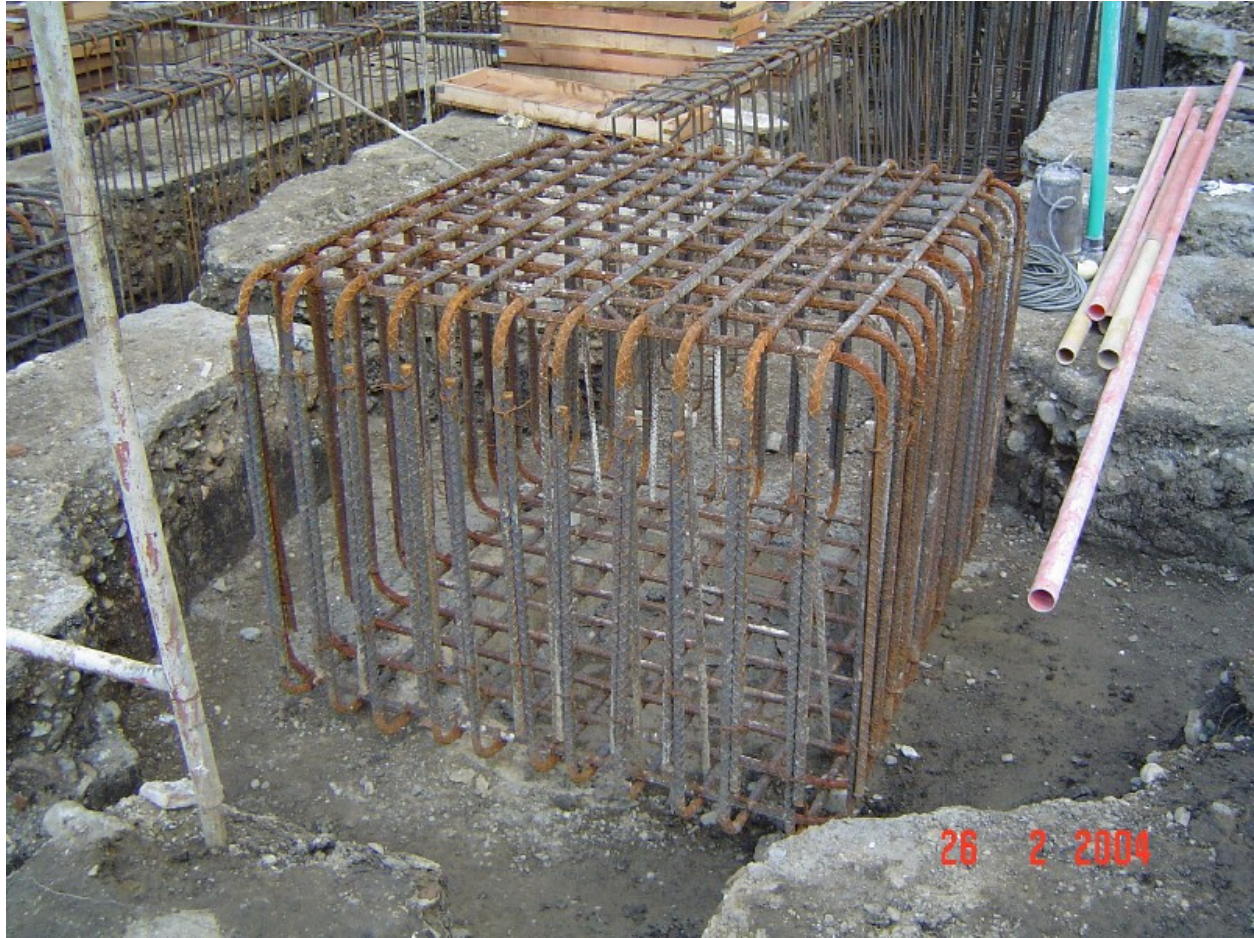
Figure 6a. Cap's reinforcement basket of a hollow pile. OPTIMA S.A. construction project.
