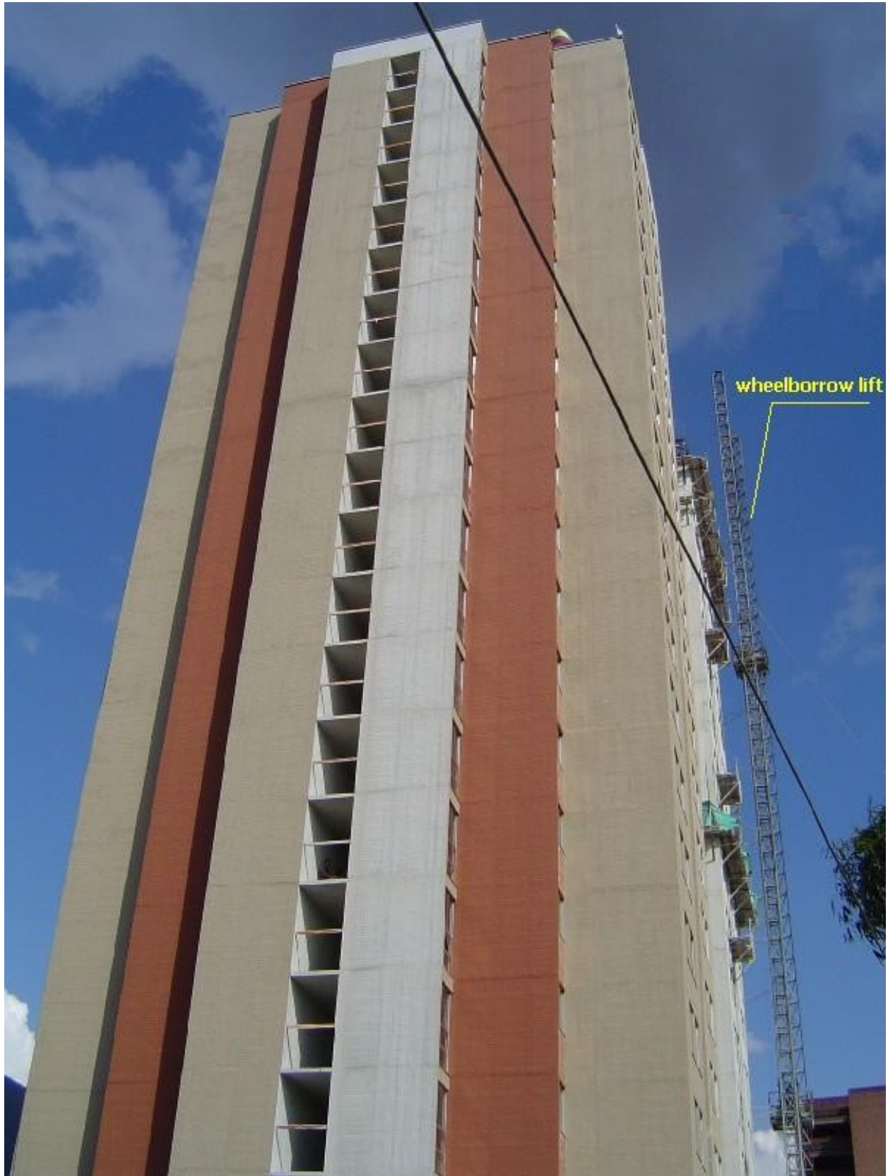
Figure 5c. Wheelbarrow lift structure to transport concrete up to high floors. OPTIMA S.A. construction
