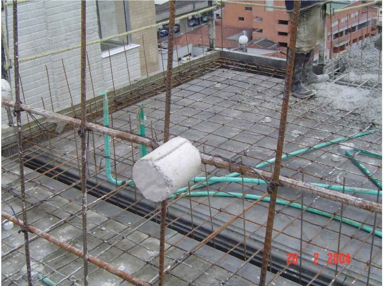
Figure 6e. Element, commonly called "panelita", used to maintain the necessary cover and to ensure the correct placement of the reinforcement into the wall. OPTIMA S.A. construction project.
