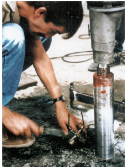
Extraction of concrete cores
