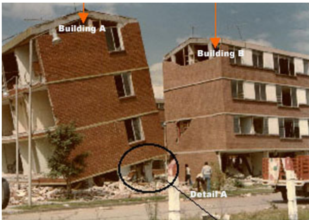
FIGURE 6D: Earthquake Damage- Inadequate longitudinal and transverse reinforcement (note the collapsed first story)
