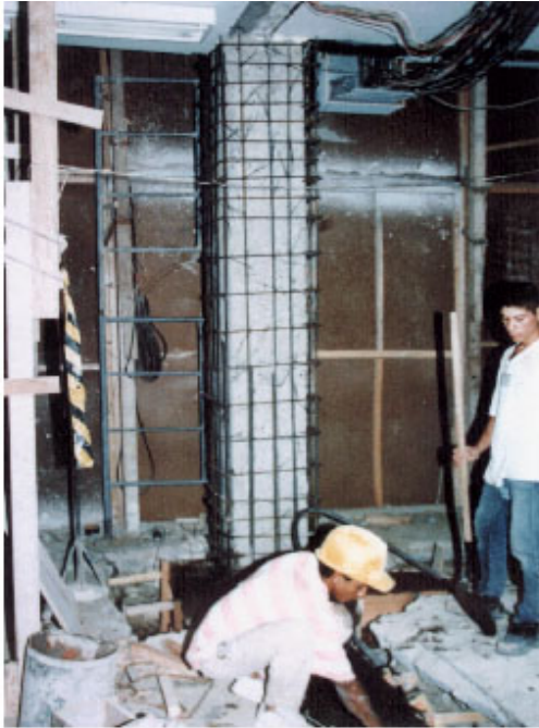
New added longitudinal and transversal reinforcement
