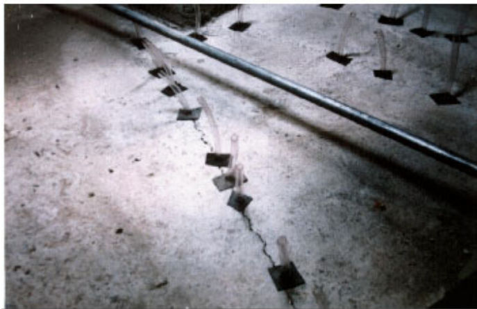
Epoxy injection of the cracks
